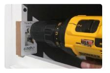
2. Screw the post into the pilot hole with the larger, #8 x 1" screw packaged with the false front kit.
