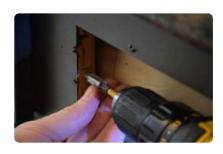
3. Screw the provided clips into the false front with the 5/8" screw in the false front kit. Look for the prepared location mark.
