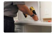
moldings of the drawer front, not the center panel. You will use these holes to attach the front to the box in step 4.
