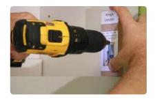
2. For a ½" overlay door, rest the door on the hinge locator block and screw the hinge to the cabinet frame. Use the ¾" washer-head screws.
